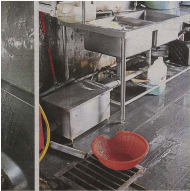
The grease traps placed under the sinks ensure food waste, grease and oil do not flow into the river.
